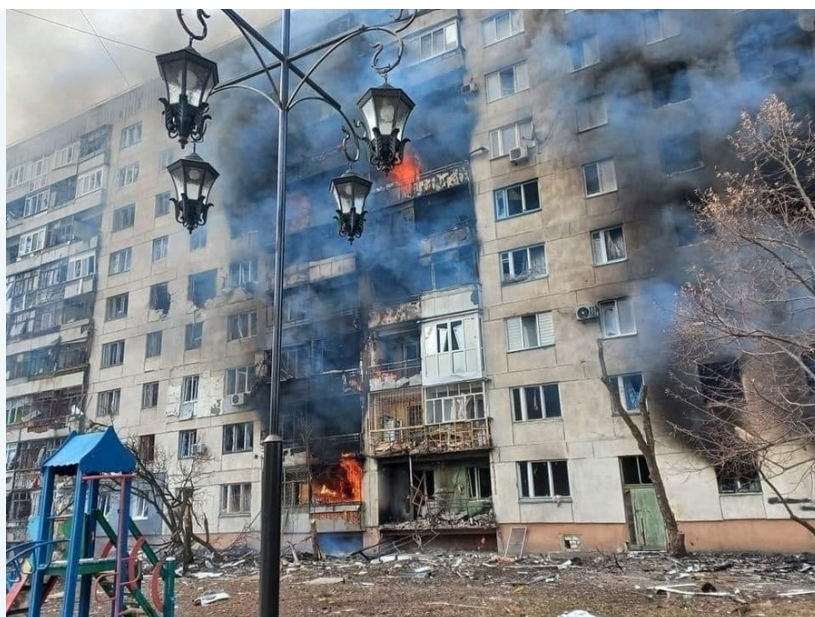
DESTRUCTION OF CIVILIAN INFRASTRUCTURE IN LUHANSK REGION © IOM UKRAINE 2022
